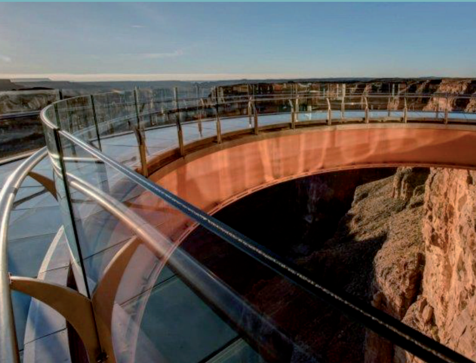
Figure 10.7. Skywalk Bridge at the Grand Canyon West (USA). Source: © IYOG archive.
