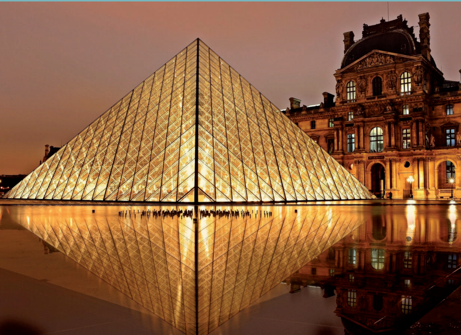
Figure 10.7. Glass buildings and structures around the world presented as candidates of the 7GW. Louvre Pyramid (Paris, France). Source: © IYOG archive.
